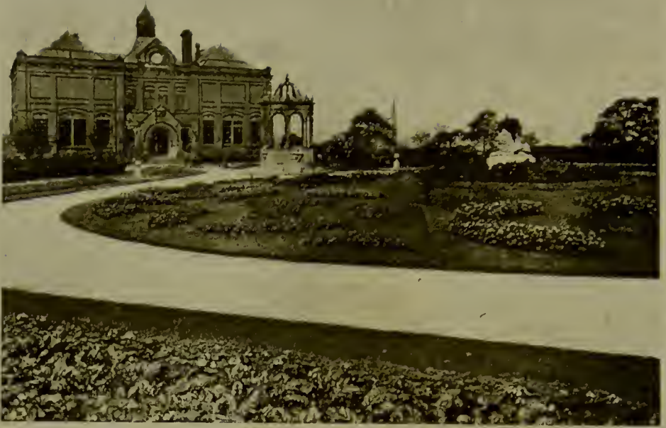
Photo by A. E. Bradburn,
